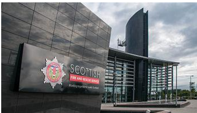
Figure 1 The Headquarters of the Scottish Fire and Rescue Service in Cambuslang, Scotland.
